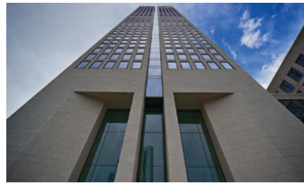
OPERA TOWER FRANKFURT, GERMANY
